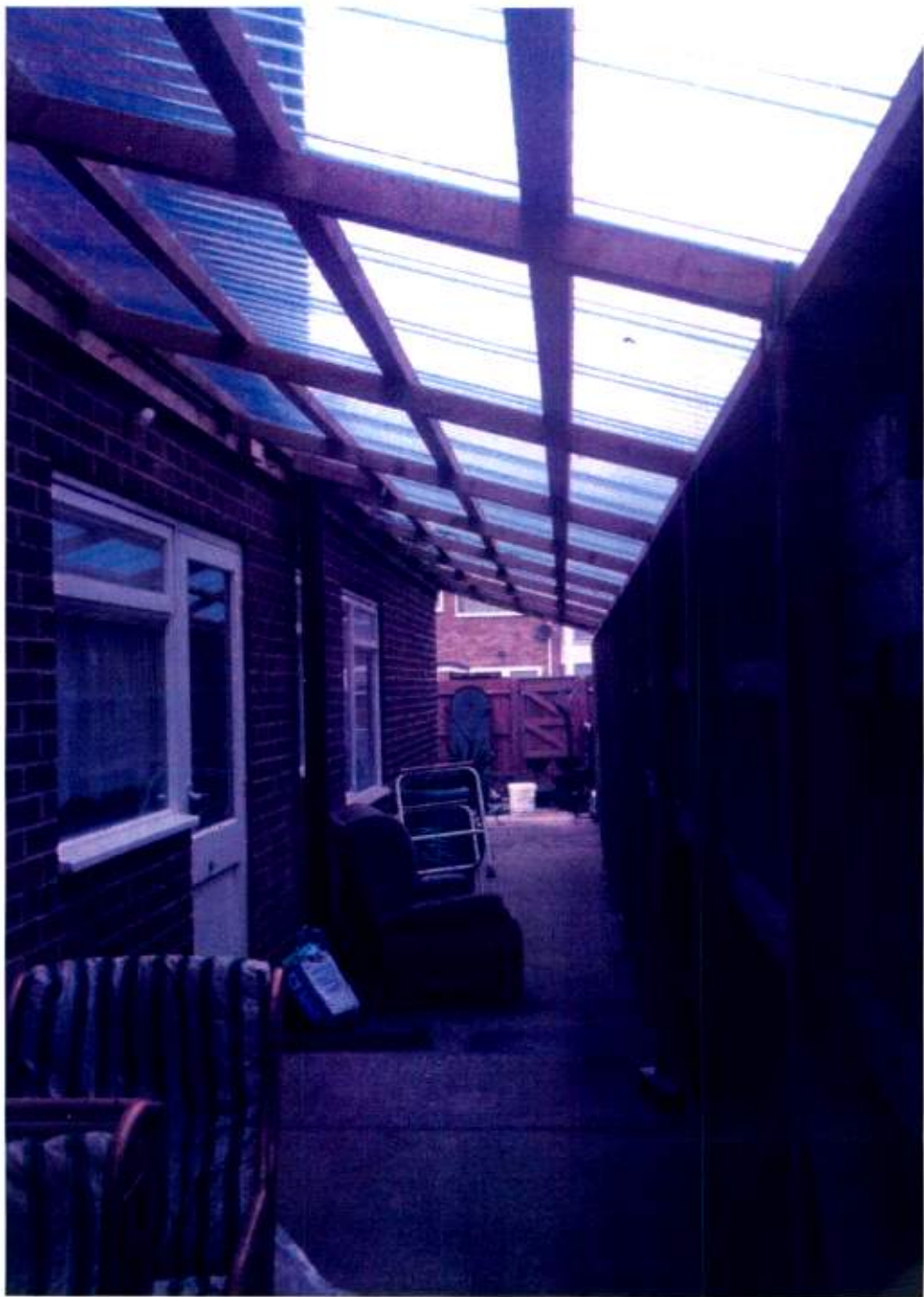
Covered area looking towards gate
