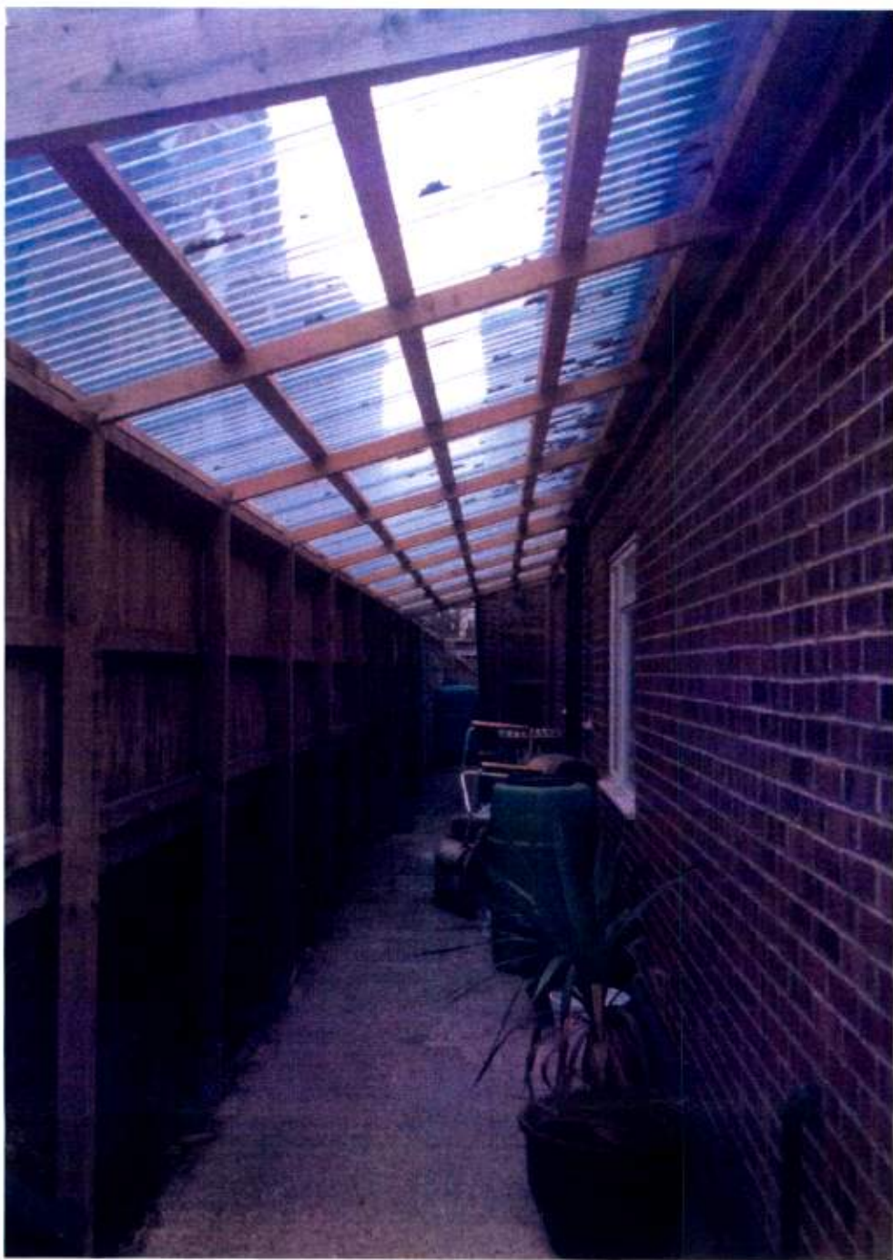
Covered area looking toward double gates
