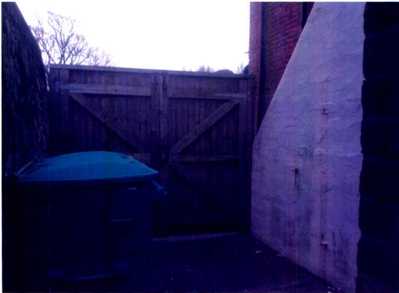
ARUN DISTRICT COUNCIL LU/82/12/DOC Sewage double gates looking from covered area
