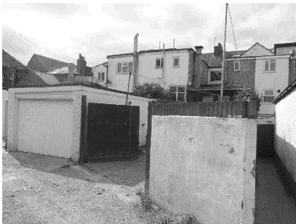
5 – Rear of adjacent Pier Road properties with The Nelson to the left
