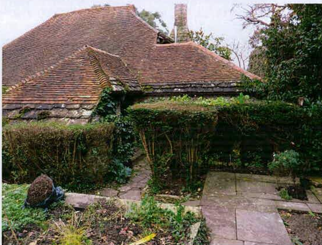
POSITION OF PROPOSED EXTENSION TO THE RIGHT WITH EXTENSION TO BE REMOVED TO THE LEFT.
