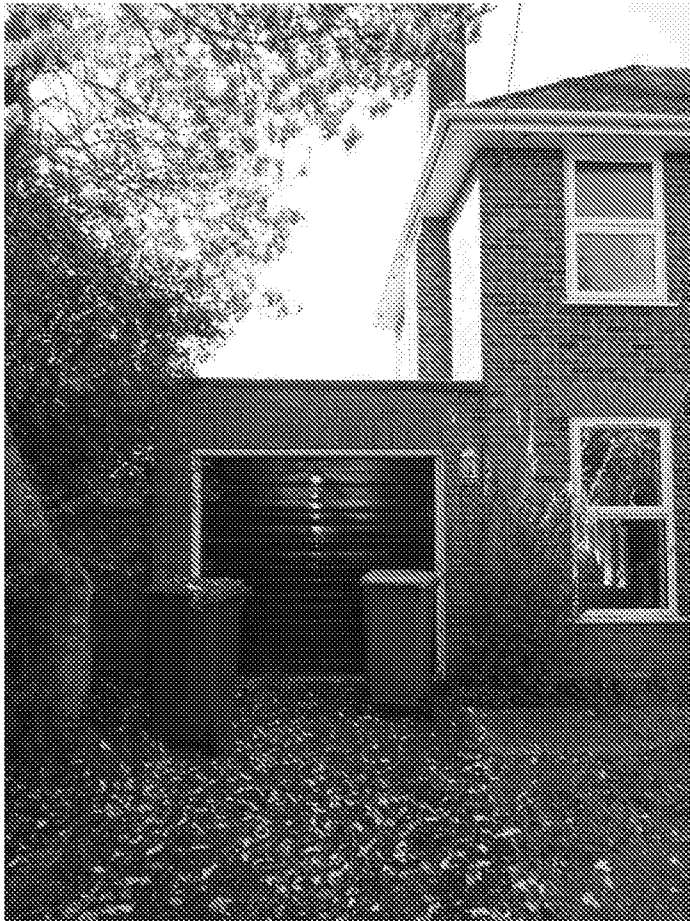
Existing garage (North facing)
