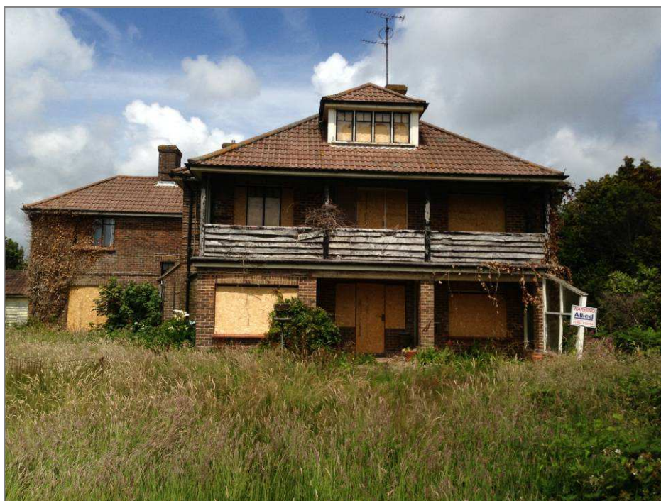
Figure 1 – South side elevation of the existing house
