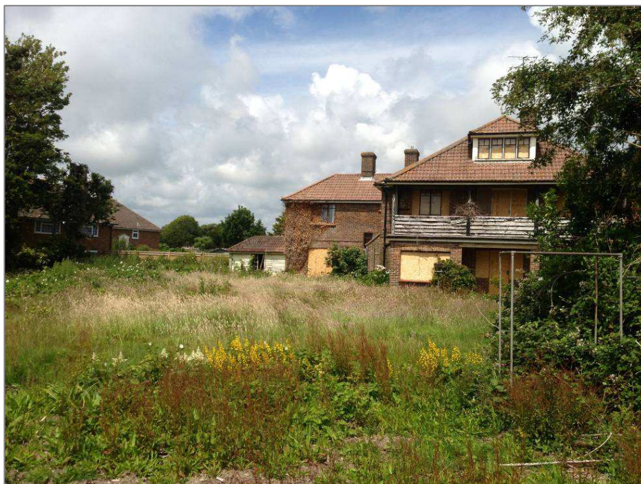
Figure 2 – Internal view looking north of the application site
