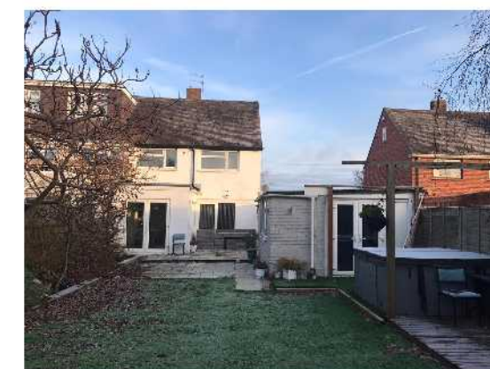
CURRENT CONDITION. REAR ELEVATION. PHOTOGRAPH DATE: 15-01-2021
