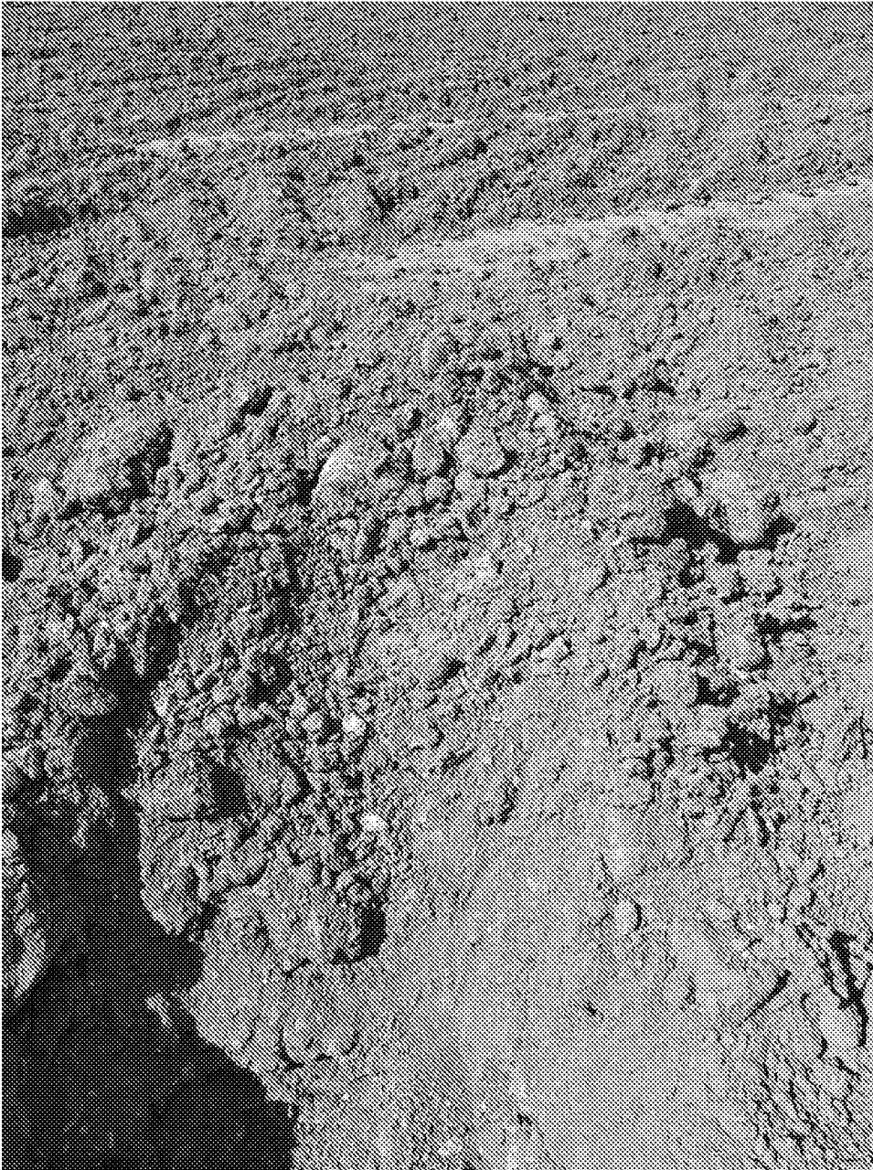
Photo of hole with tape in place
