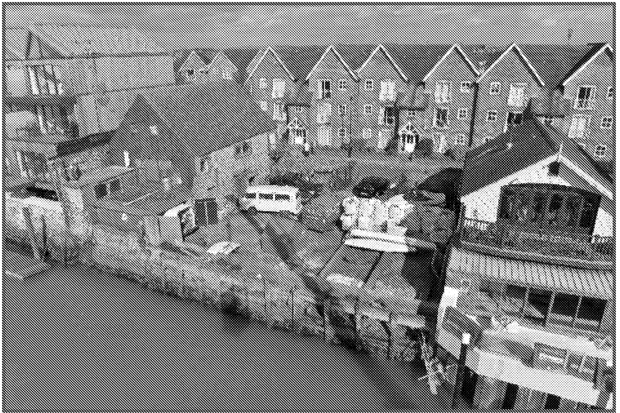
Figure 4-5 Frontage at the proposed works within Reach 4
