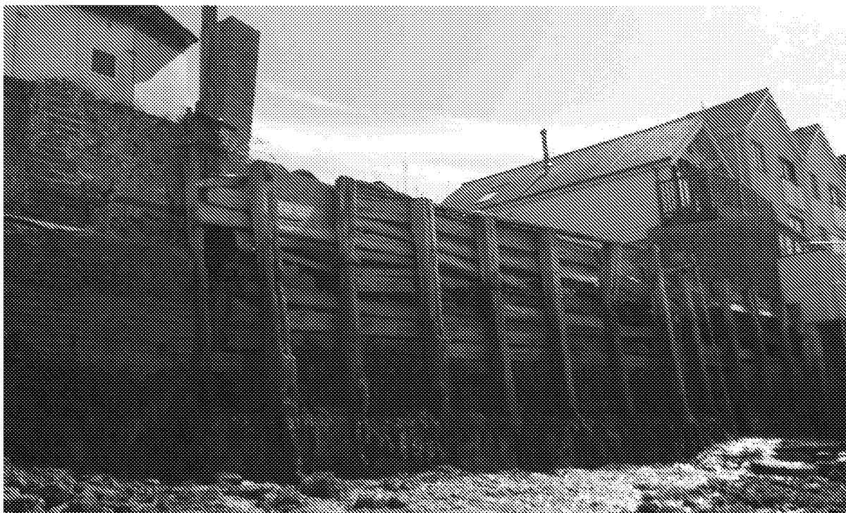
Photograph 1. Existing flood defence wall showing upstream and downstream extent of site boundary
