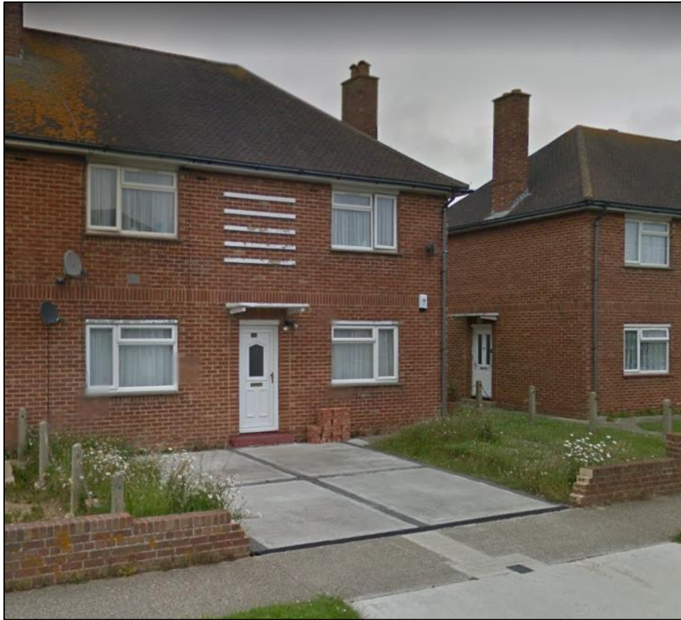
Concrete Driveway at 71 Wick Farm Road adjacent to application site
