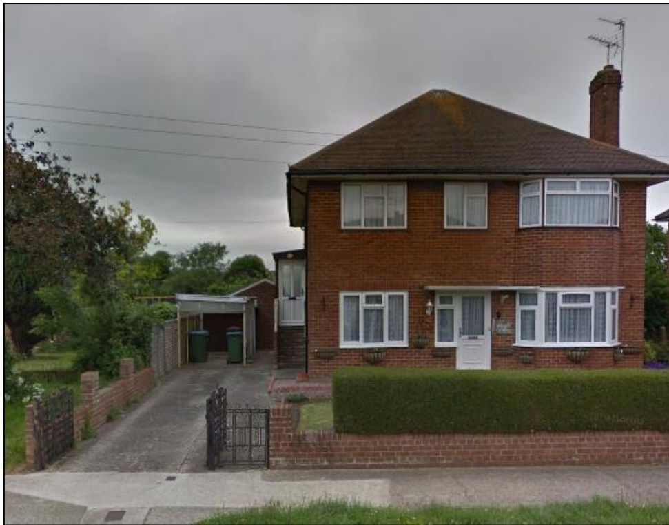
Concrete Driveway at 63 / 65 Wick Farm Road to the west of the application site
