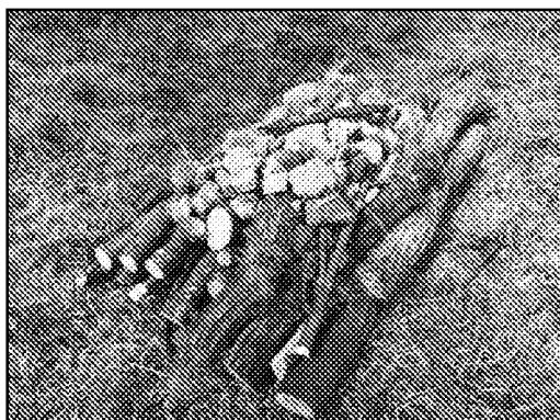
Figure 2: Unfinished log piles with rubble centre
