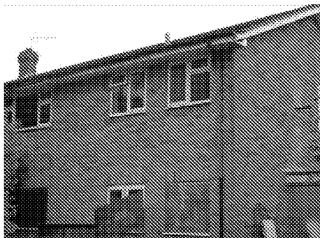
Photo 1. Northern elevation of derelict house
