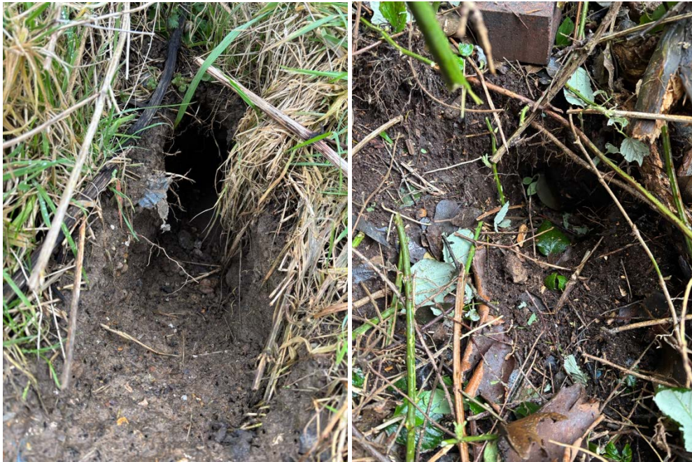
Figure 1: Shallow holes identified during the site visits
