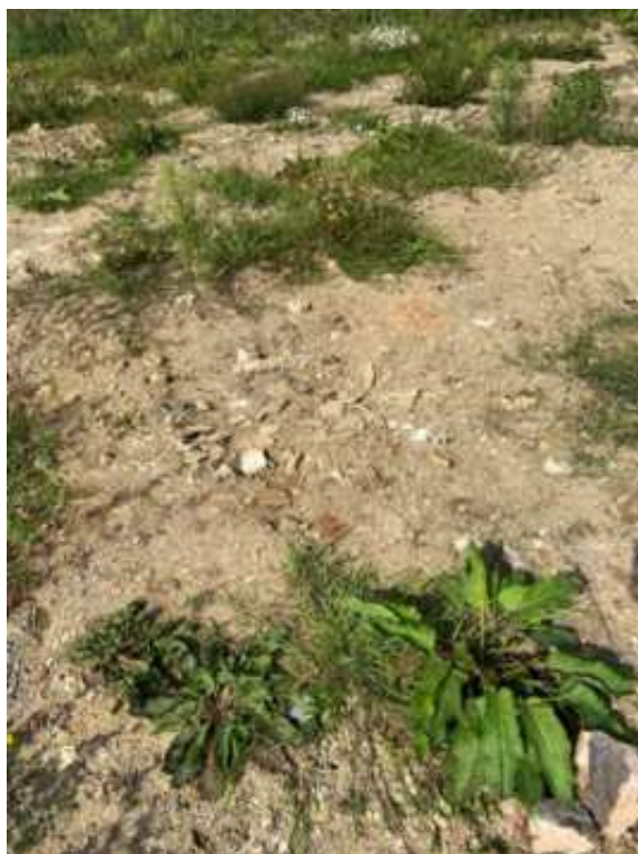
Plate 3 Crushed asbestos containing sheet at surface
