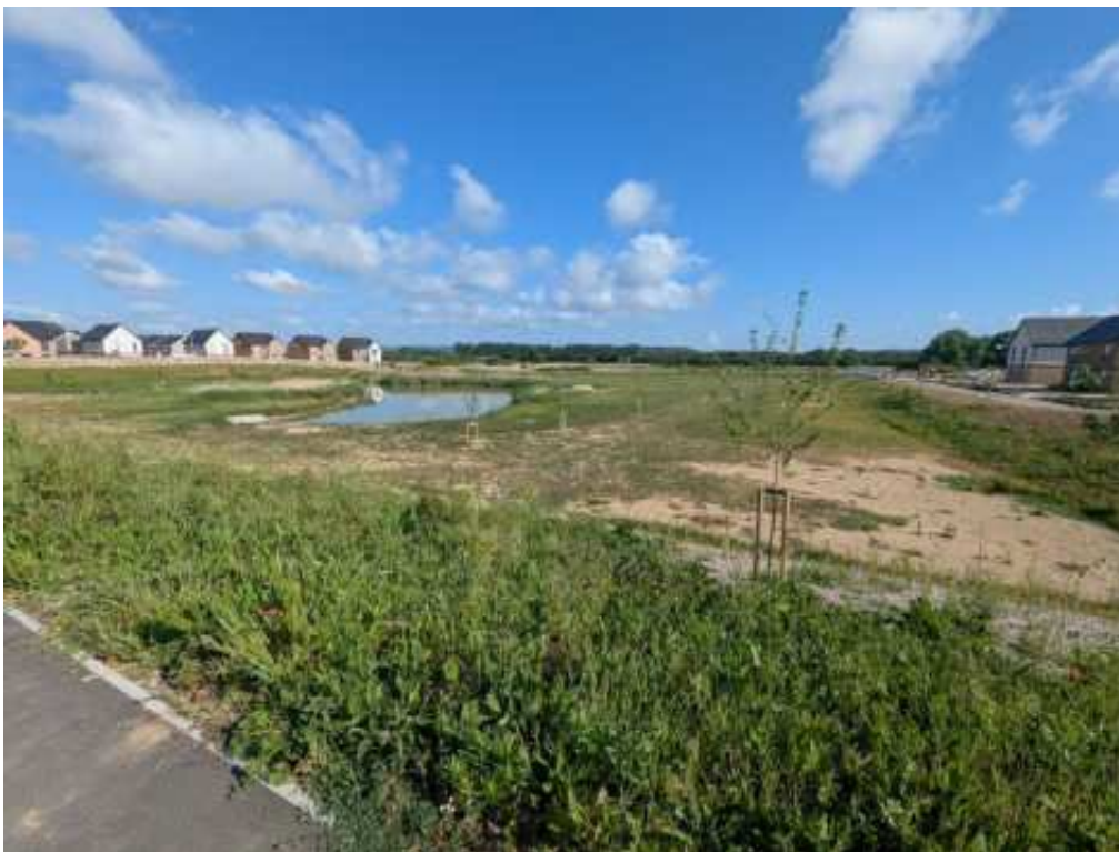
Client provided photo showing topsoil in place in the Wetlands
