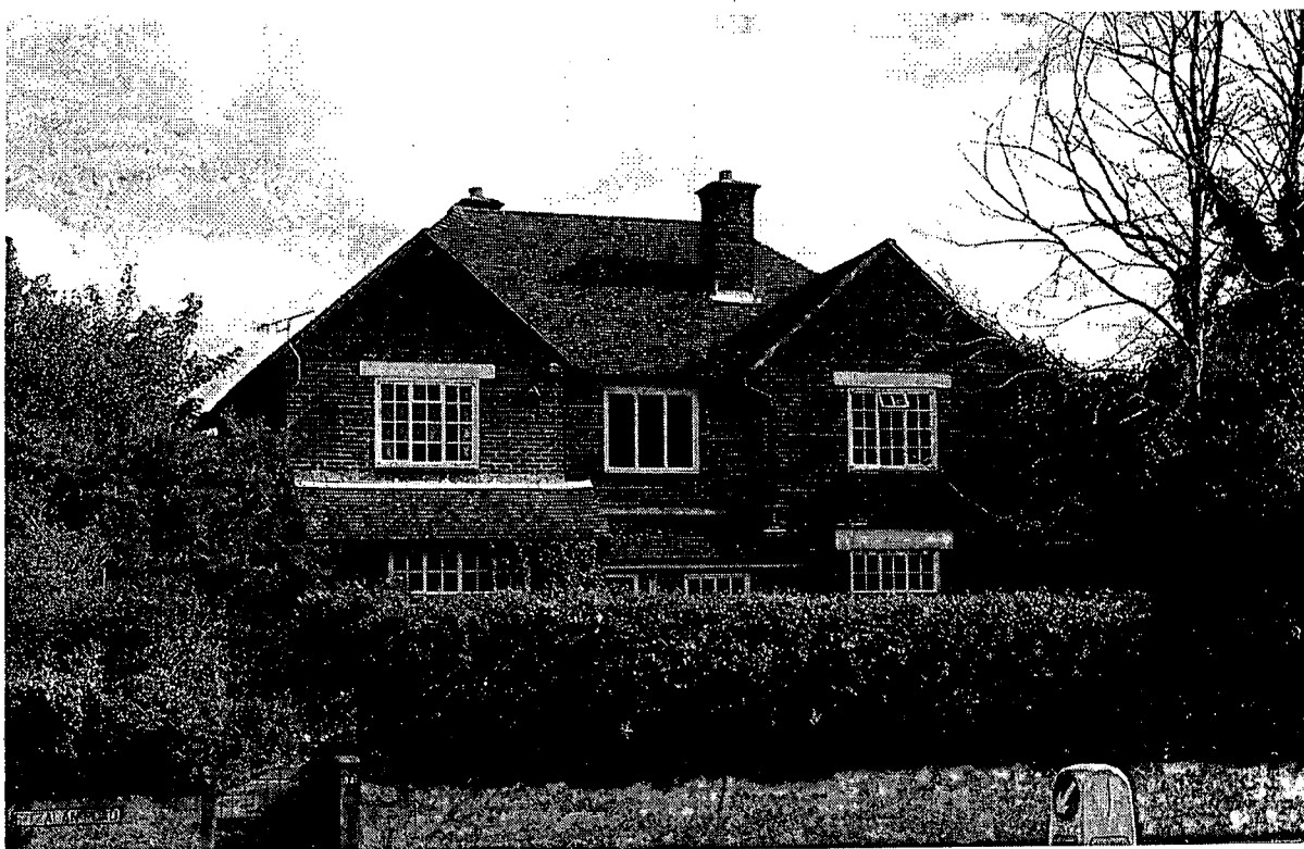
3. No. 34 Fitzalan Road ( The Vicarage) on the site.
