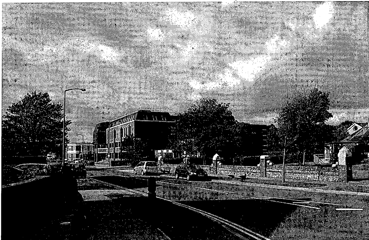
17. View west along Maltravers road.
