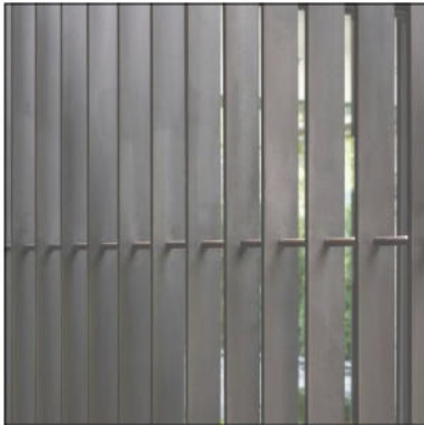
5. VERTICAL METAL SCREEN GATE PANELS
