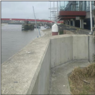
3. EXISTING STONE & CONCRETE RIVER WALL
