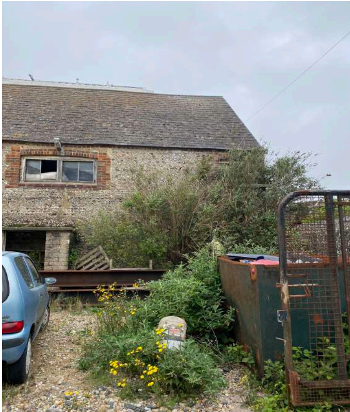
Photograph 3: The existing garage and adjacent yard area (used for vehicle parking), facing northwest.
