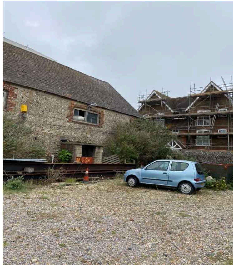
Photograph 4: The existing garage and yard area as well as neighbouring residential buildings, facing northeast.
