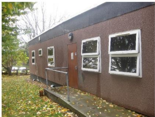
Rear fire exit
