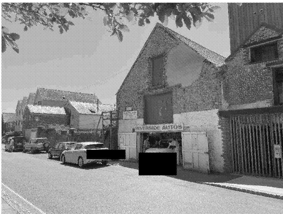
River Road frontage looking South West
