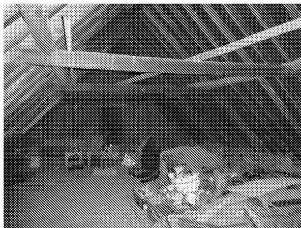
Figure 22: Collared truss roof structure
