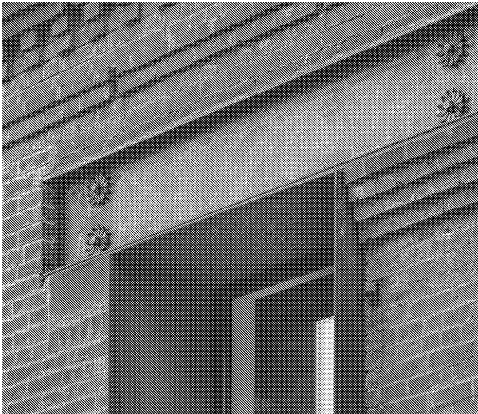
Feature lintel on historic warehouse
