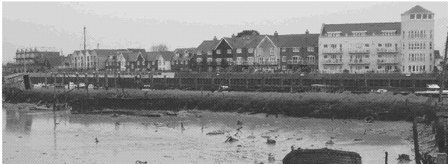
East river frontage - building heights generally 3 to 6 storeys
