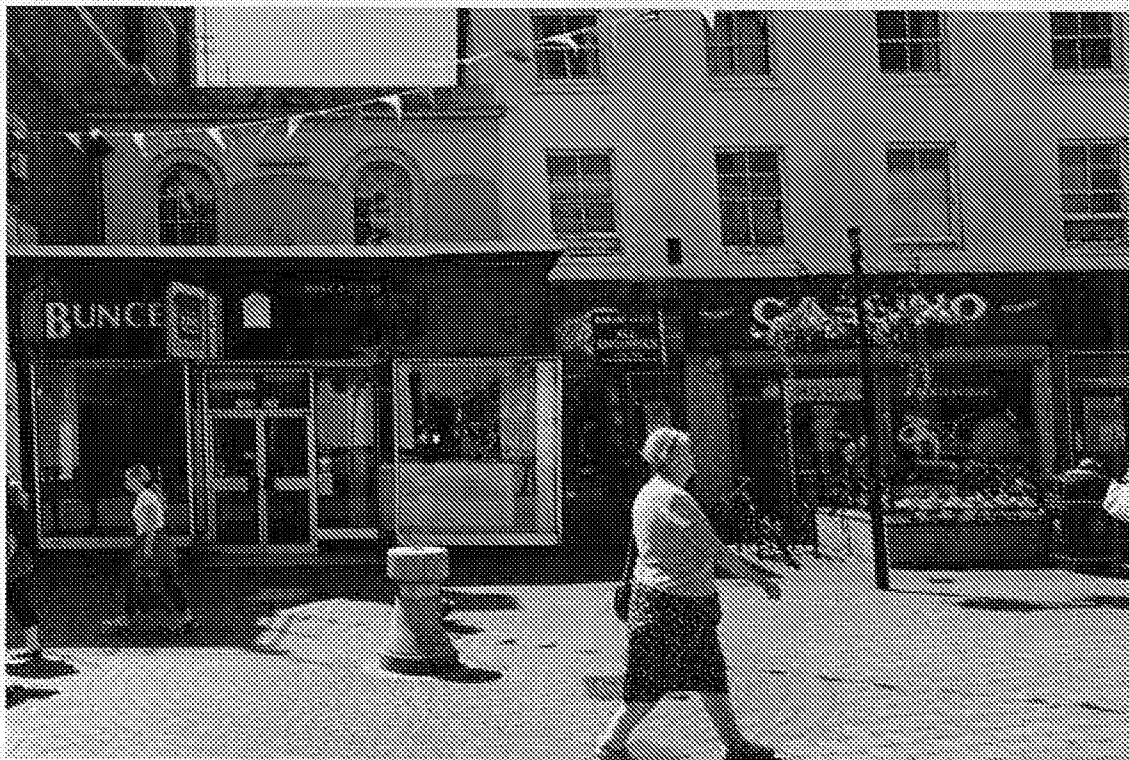
FIGURE 1: View of the building fronts on High Street (No.48 right, No.50 left)
