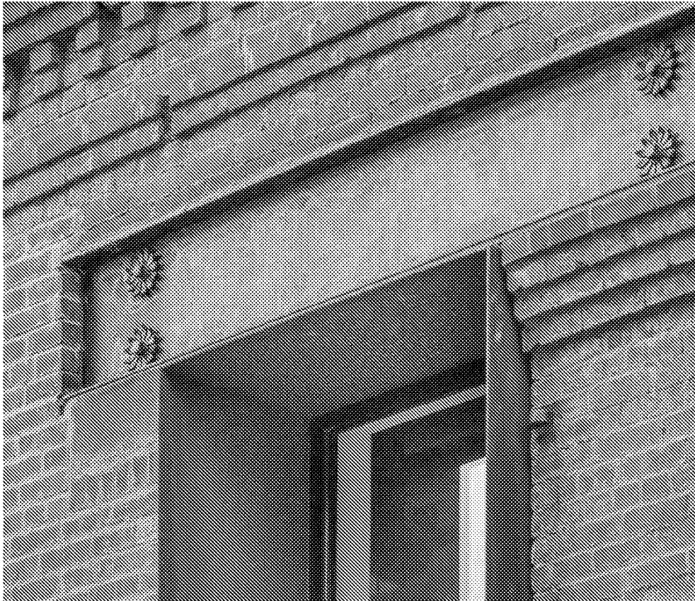
Feature lintel on historic warehouse
