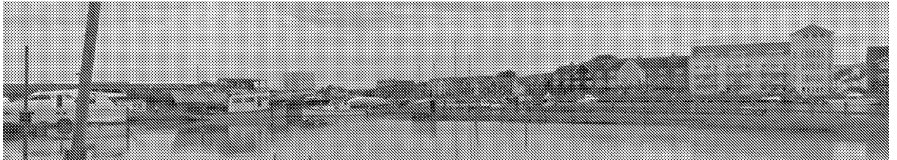
Varied skyline from the English Coast Path on the south side of the river. The Harwood Road gas holder is due to be dismantled.
