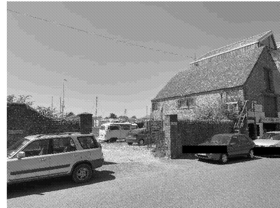
River Road frontage looking north west
