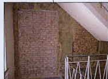
PHOTOGRAPH A BRICKED UP DOOR OPENING
