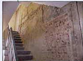
PHOTOGRAPH C GENERAL VIEW AT GROUND FLOOR LEVEL
