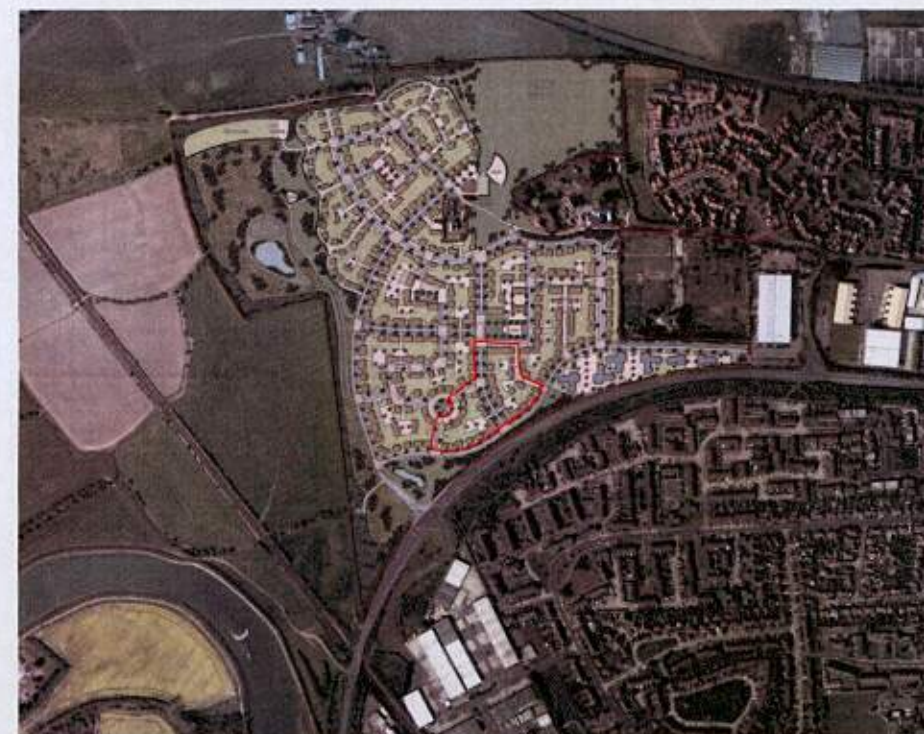
Figure 2: Aerial View with Phase 1B/2 outlined in red
