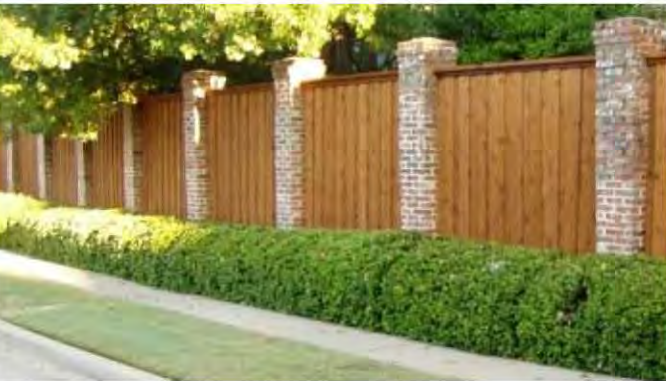
Brick piers and timber infill fencing
