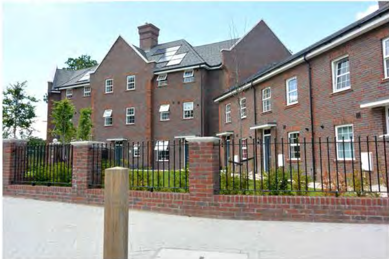
Low level railing with brick piers
