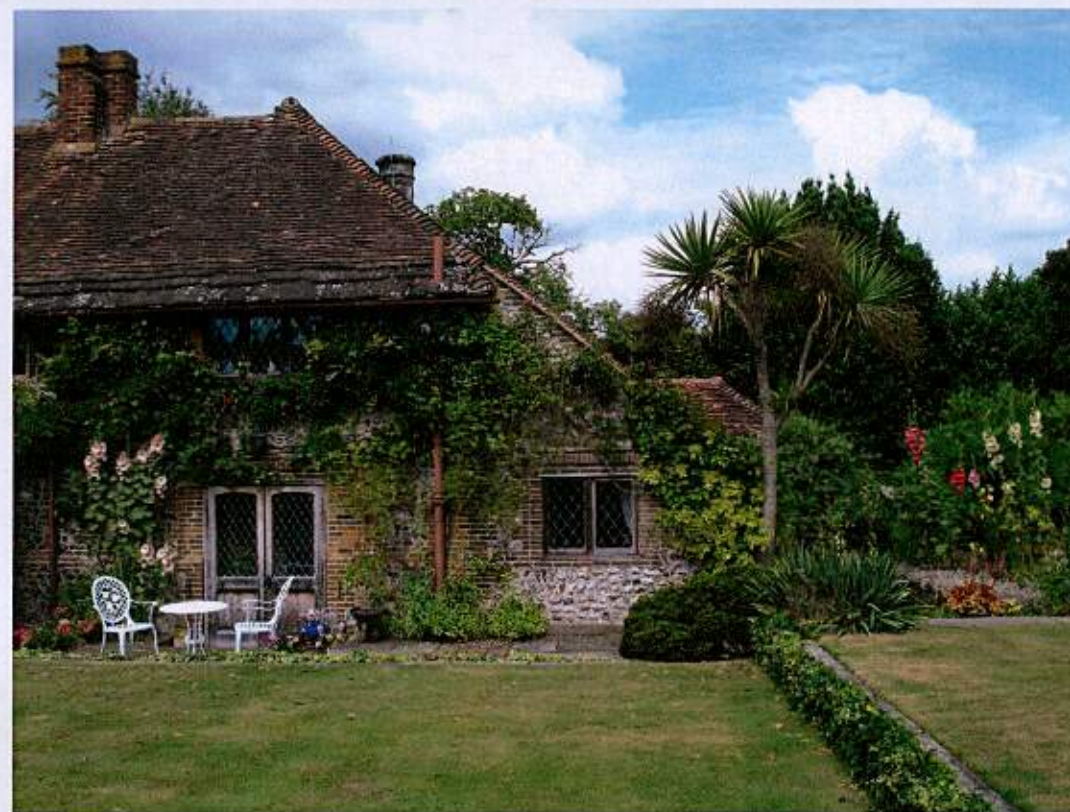
PART VIEW OF SOUTH-EAST ELEVATION WITH LATE SMALL EXTENSION TO BE REMOVED IN THE DISTANCE ON THE RIGHT HAND SIDE.
