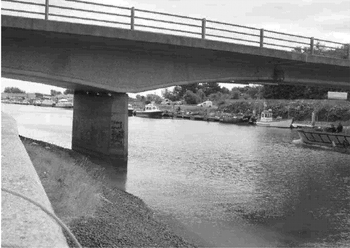
Plate 34. The bridge at the far southern end of the Site, looking south towards the moorings of Littlehampton Marina and industrial zones.
