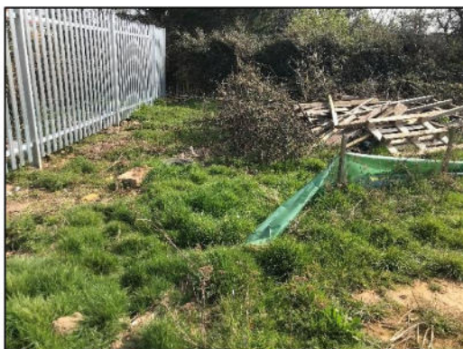
Figure 12: Destroyed reptile fencing along the northern boundary
