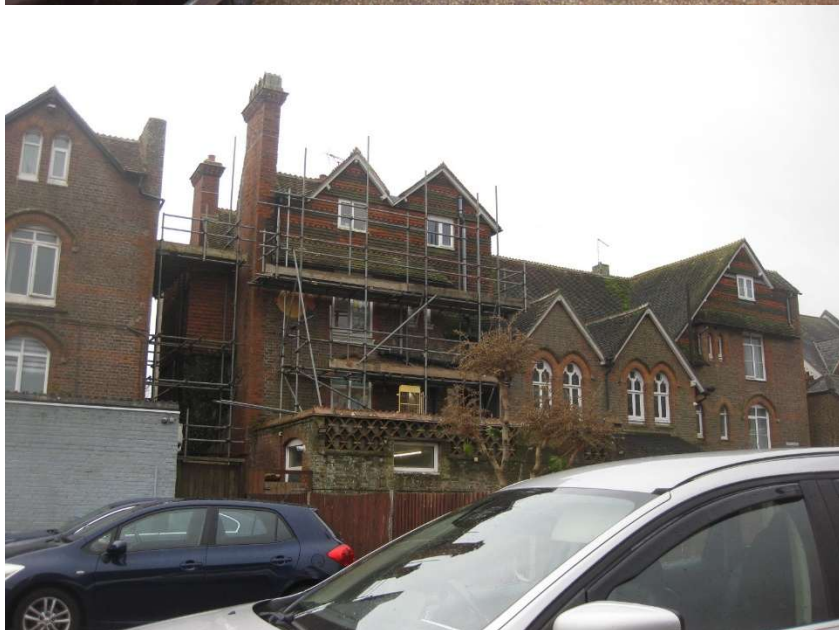
5 Selborne Place (partly with scaffolding) viewed from Selborne Road looking south.
