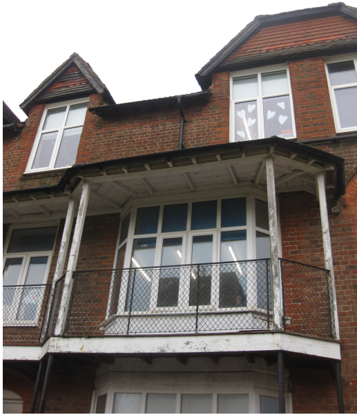
Balcony - floor above the extension to be removed and replacement timber posts installed
