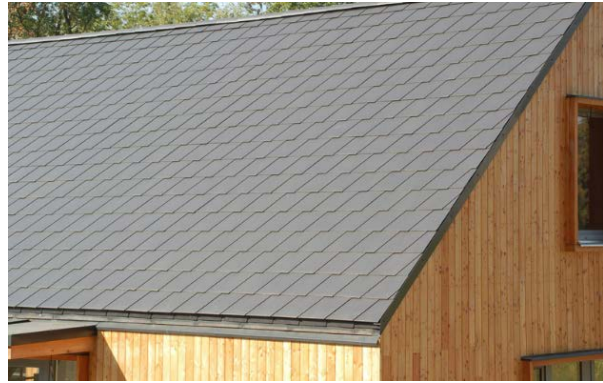
Two examples of the Jutland slate tile.
