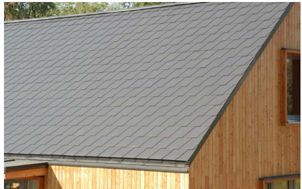
Two examples of the Jutland slate tile.
