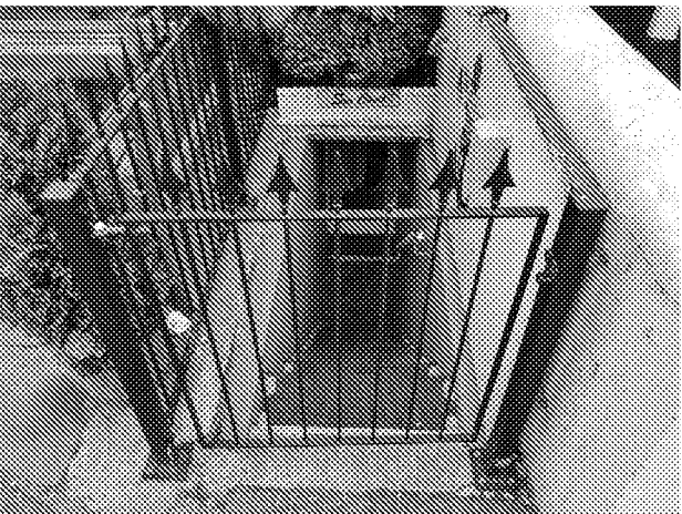
Photograph of existing railing style, to be continued in proposal
