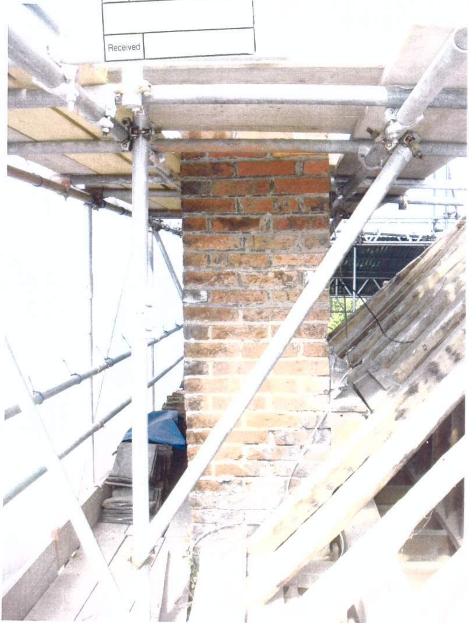
BASE SECTION OF CHIMNEY NO. 3
