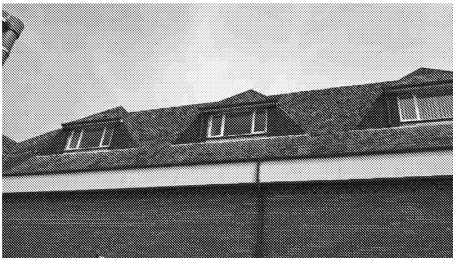
Plate 2 – View of the dormer windows present on the second level of the south facing side of B1.
