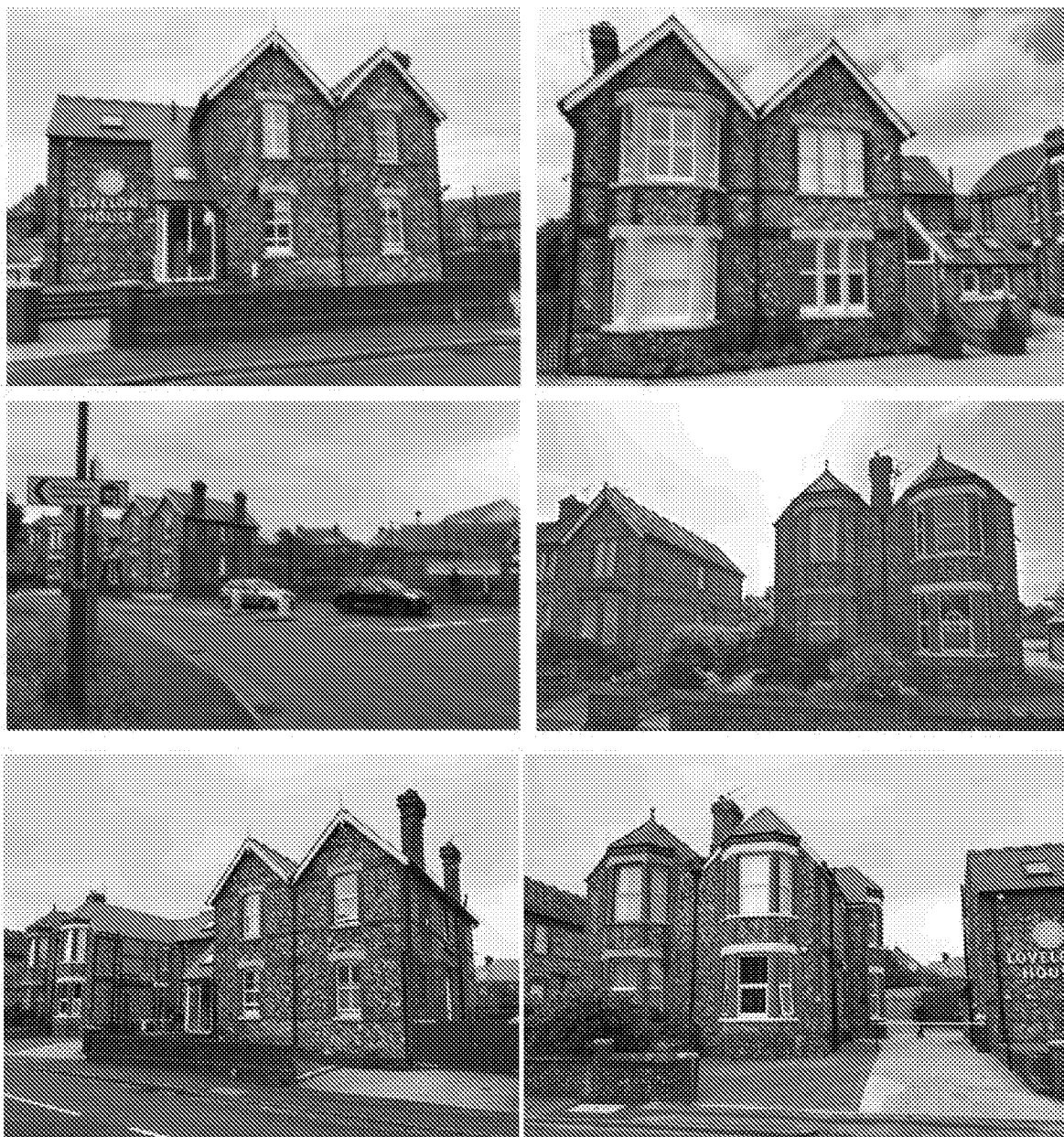
Figure 2 Street Views of Site
