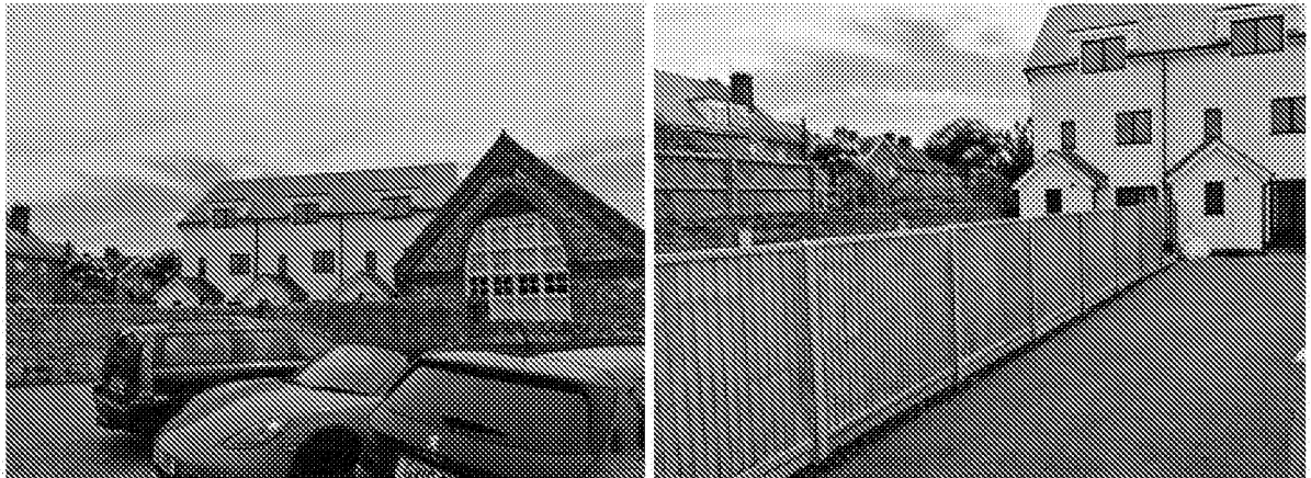
Figure 3 Views of recently completed former Dairy site to rear
