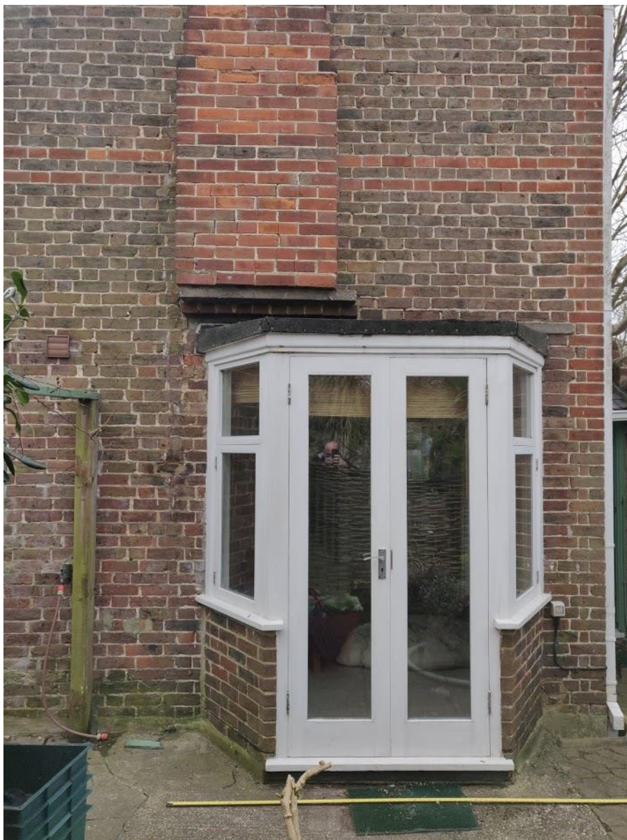
View of 11a Irvine Road from the north/rear garden showing later bay extension with doors to be removed.
