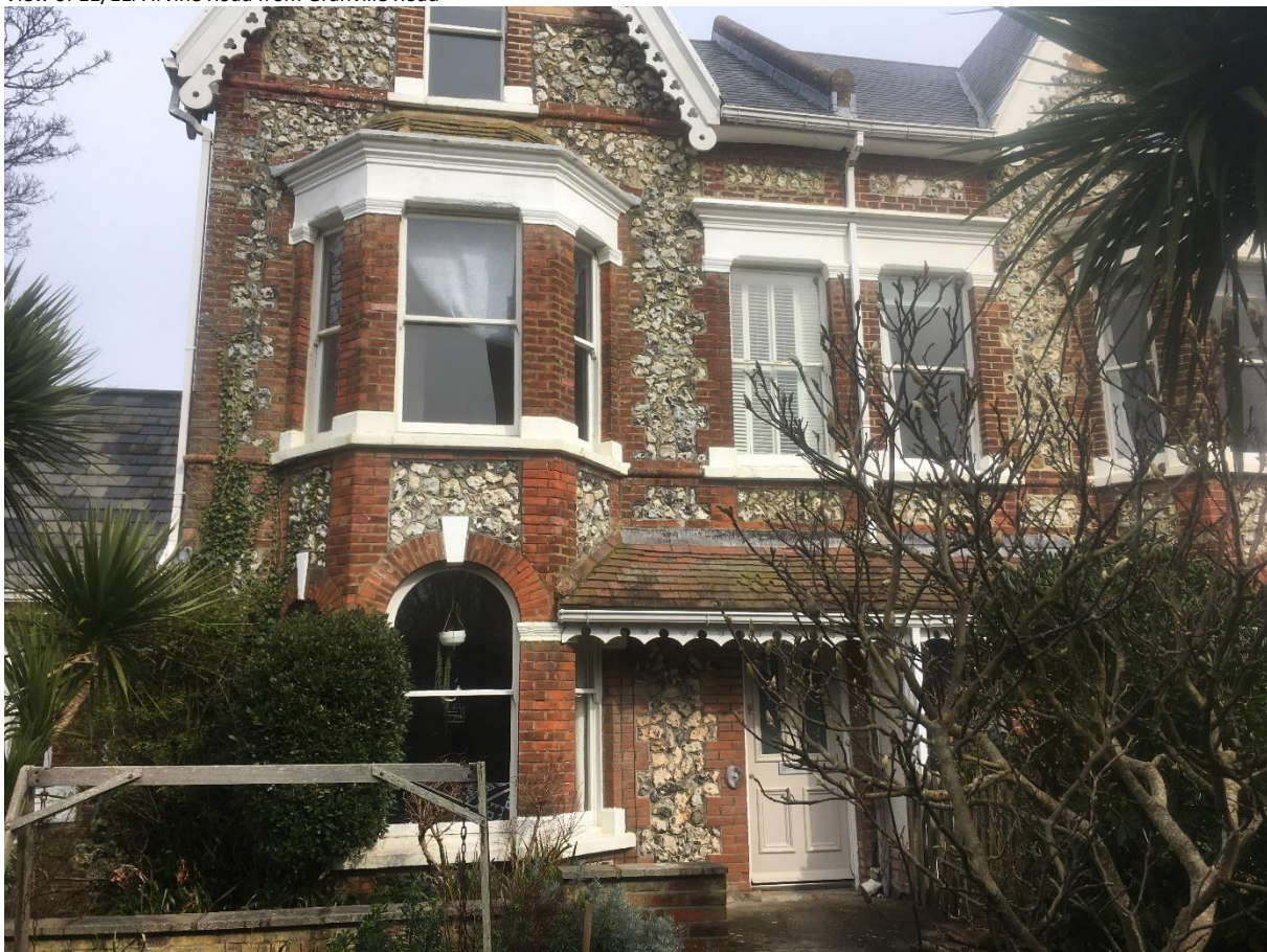
View of 11 Irvine Road from the south and front garden
