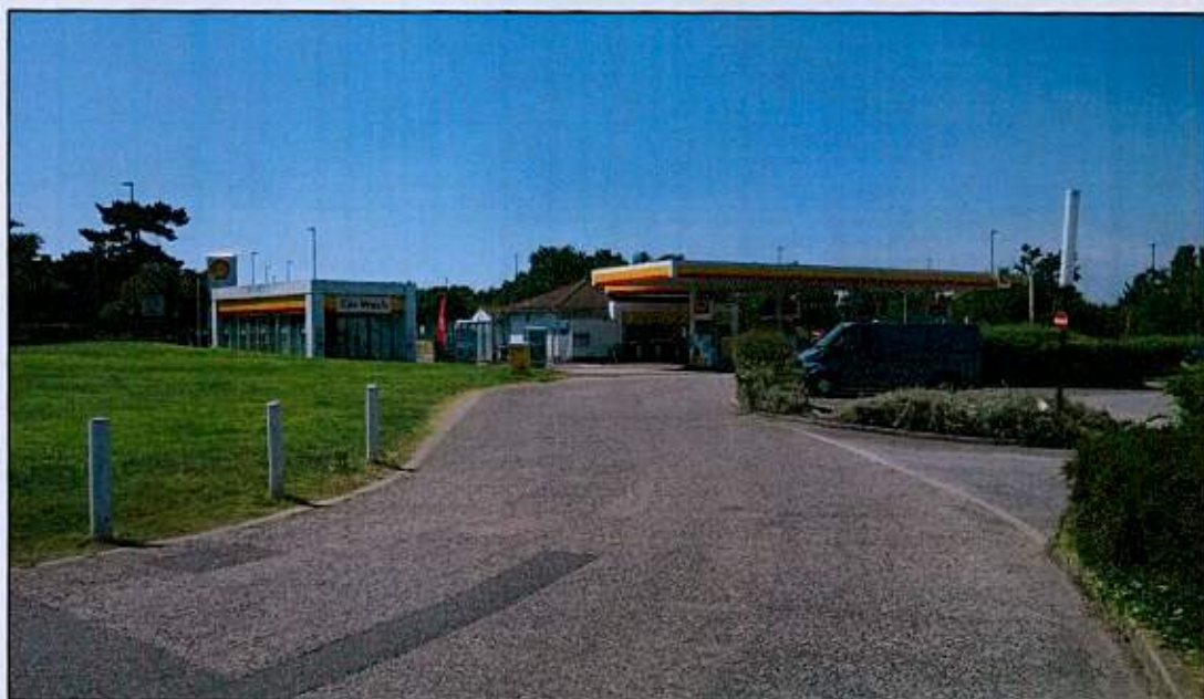
Figure 3.1: Existing Access Road
