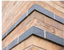
Brick Detail Contrasting Blue Brick example
