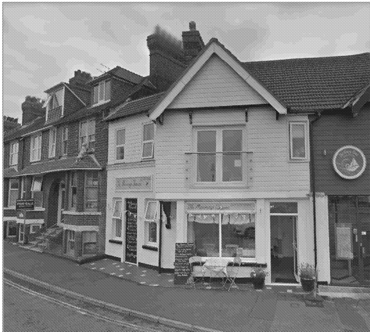
Figure 2: View of the site from Pier Road to the west (Source: Google Streetview)
