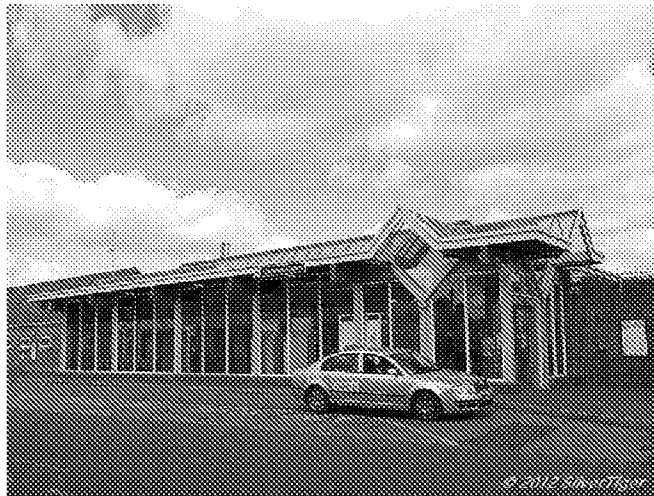
Photograph 7: Littlehampton Railway Station
