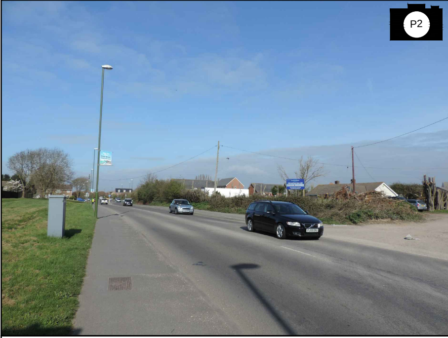
P2: Looking at the site frontage from Worthing Road. Hedge 16 is in generally poor condition with dead sections. Where viable, it will be retained and reinforced with new landscaping.
