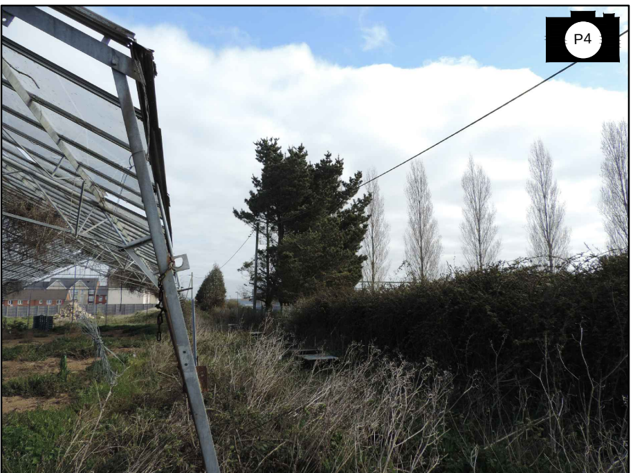
P4: Trees 2, 3 and 4 grow on the adjacent site. They have been regularly cut back from the overhead power cables resulting in asymmetric crowns and poor form. They have little long term potential.
