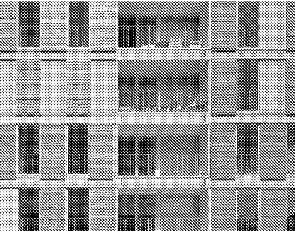
Variable privacy and sun screening for large-surface façade designs.
