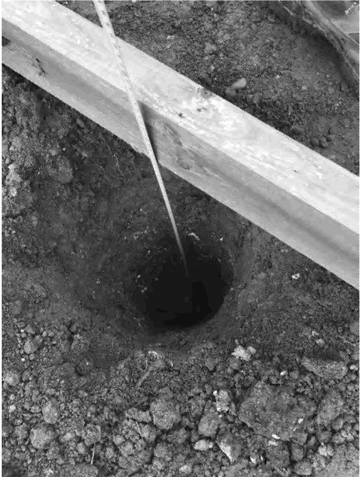
Plate 3 – Photograph with tape in place showing inspection pit dug in Plot 23
