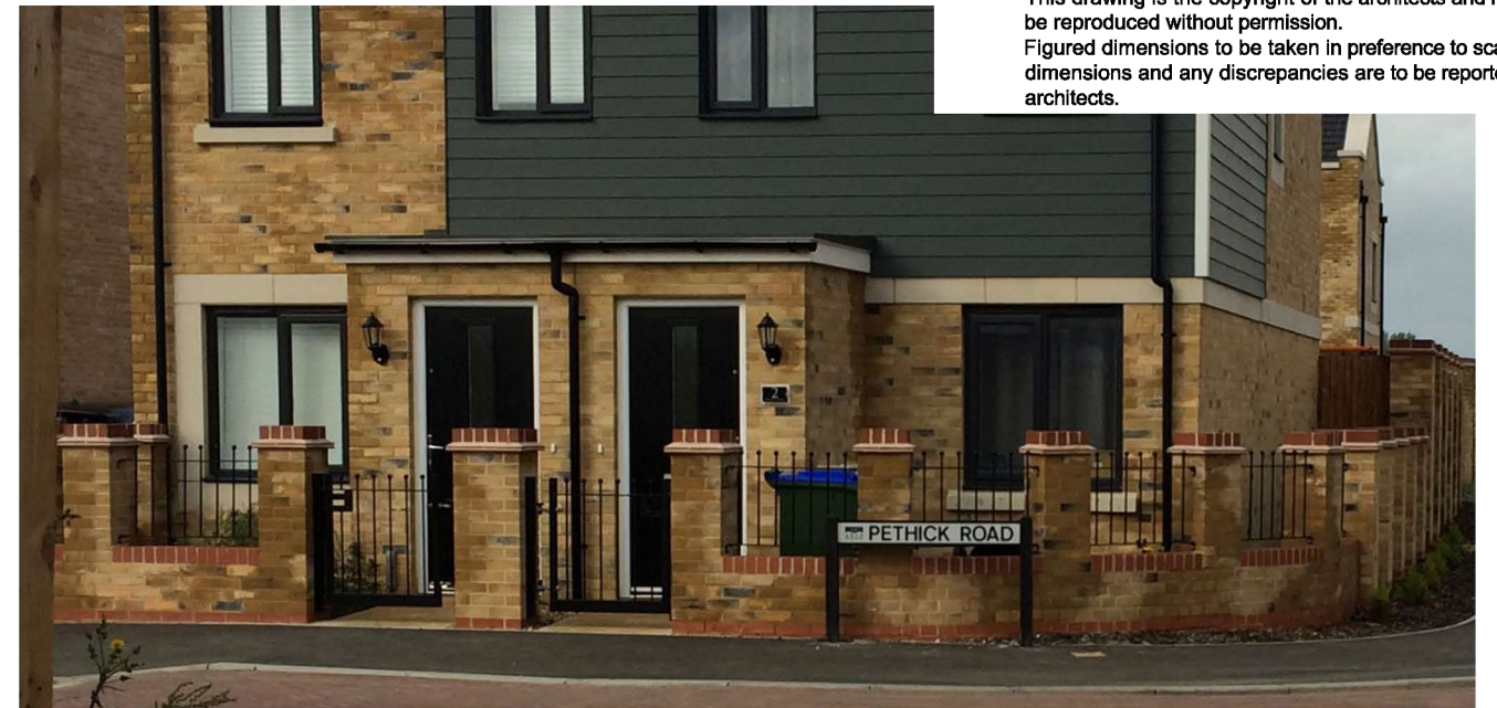
BOUNDARY TREATMENTS : Low Level Wall with Brick Piers & Metal Rainings
