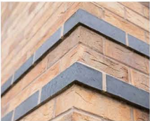
Brick Detail Contrasting Blue Brick example
