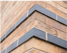
Brick Detail Contrasting Blue Brick example
